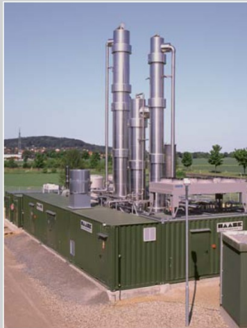
Above: The BiogasUpgrader in Jameln has been refining 100m 3 /h of raw biogas to biomethane for the local Raiffeisen petrol station since June 2006.
